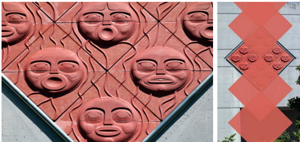
Figures – Example of smaller precast panels in diamond orientation with integrated pigment and rounded embossing (left) and conceptual example of potential pattern (right)
