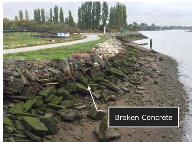
Existing concrete at Musqueam's foreshore, used for erosion protection ("riprap"). This will be replaced by erosion protection made of rock. Photo provided by Core Project Management.
