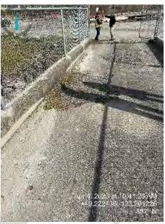
Photo 3-6: Damaged portions of Musqueam pier.
