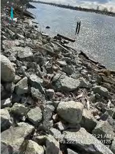
Photo 3-5: Portion of bank armouring with engineered riprap looking east from access road.
