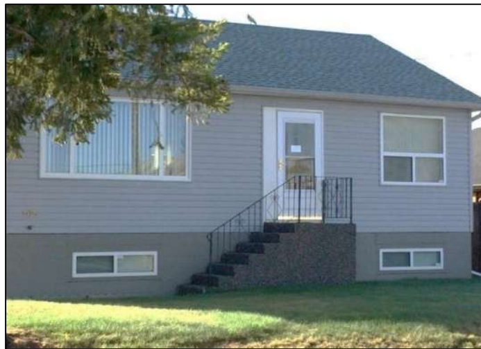
Figure 2. For this house, the Setback from the property line is measured from the house, while the steps leading to the front door are in the Setback area but do not count for the measurement.
